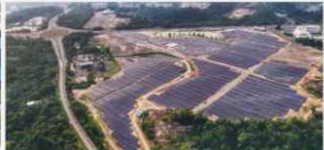
30MW AC Photovoltaics Power Plant
